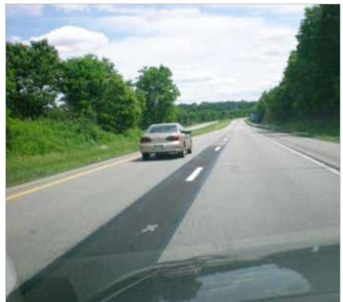
*Patching of the longitudinal joint extends pavement life.*
