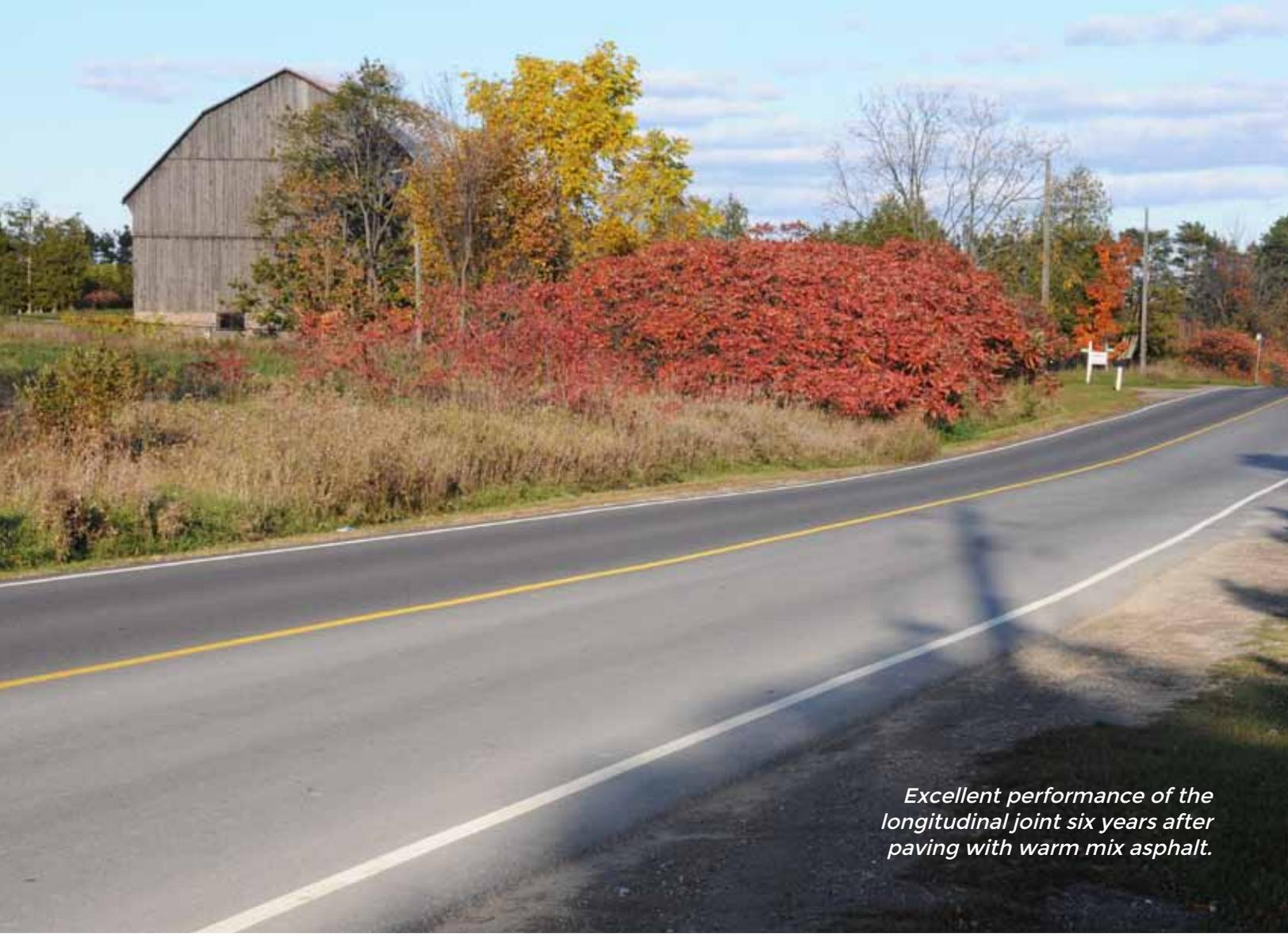
*Excellent performance of the longitudinal joint six years after paving with warm mix asphalt.*
