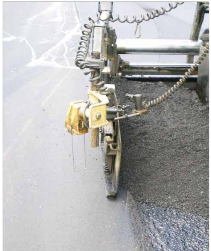
*End gate all the way down and proper overlap.*
